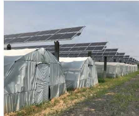
Fig. 45: PV modules above a polytunnel © BayWa r.e.
