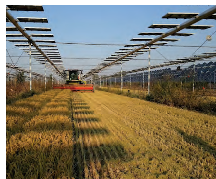
Fig. 48: Stilted, overhead systems with narrow PV modules in Italy © REM Tec
