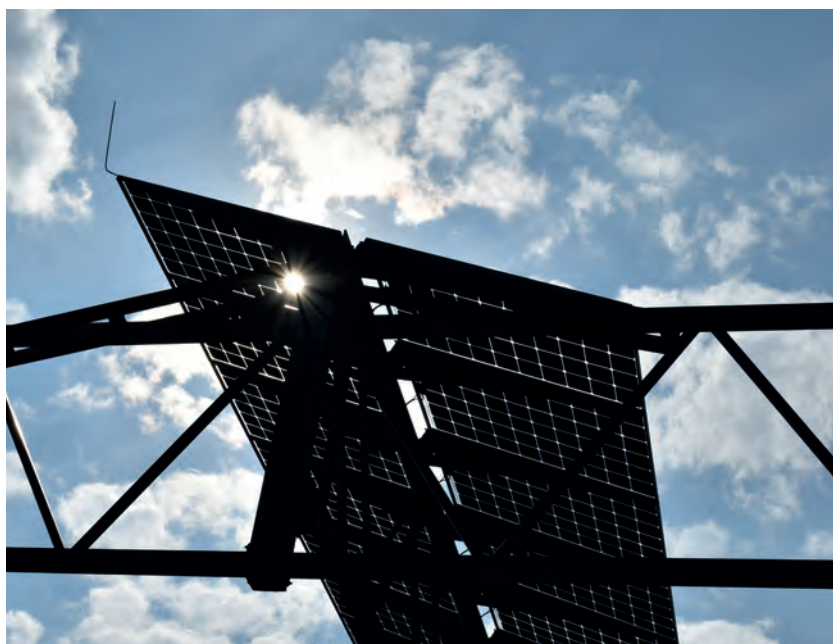
Fig. 19: Module row with bifacial PV modules on the agrivoltaic system in Heggelbach © Fraunhofer ISE
