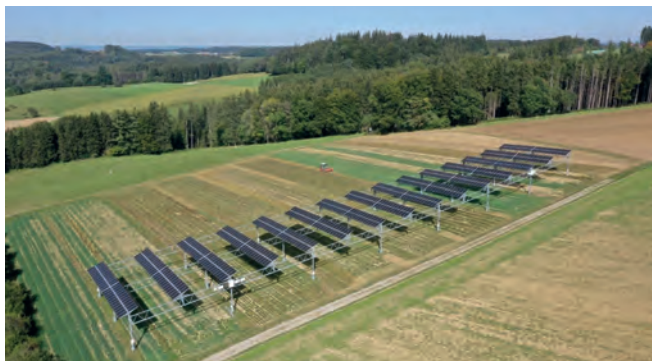
Fig. 56: Agrivoltaic system in Heggelbach with a capacity of 194 kW p , covering approximately a third of a hectare © Fraunhofer ISE
