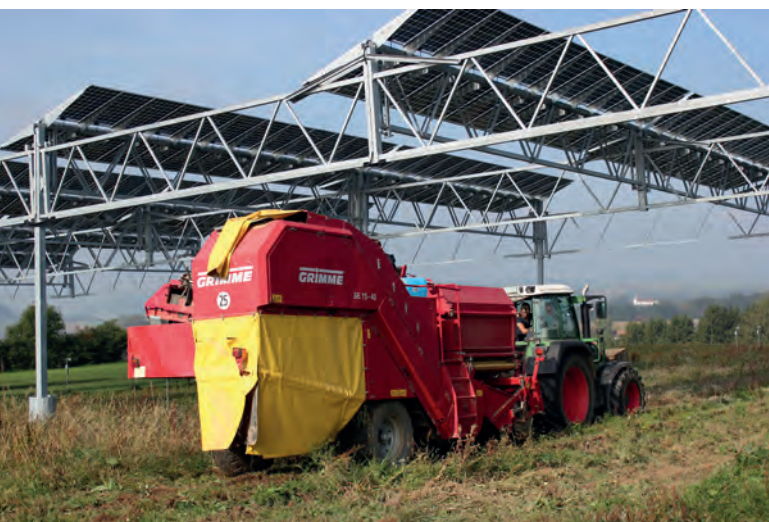
Fig. 42: Stilted, overhead system enabling cultivation with a potato harvester © Hofgemeinschaft Heggelbach
